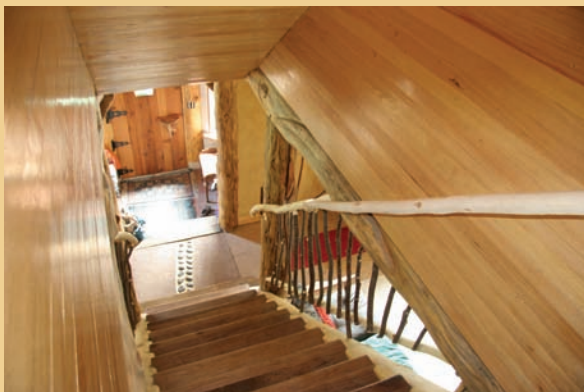
The stairway is lined with 2 1/4" oak flooring from their first home and has aspen handrails.
