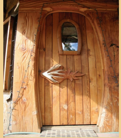
Front door made out of 4"x 4" beams, stained glass window and elk antler door knob.
