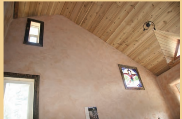
The ceiling is 1"x12" cedar and pine siding from ReSource.
