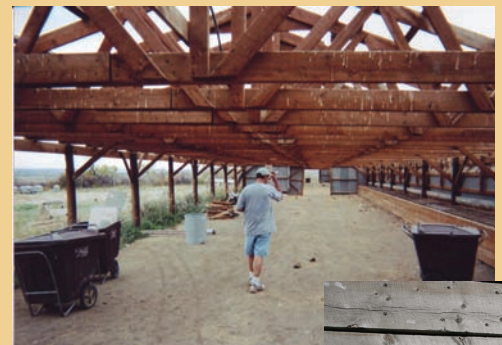
Before: Schooley Turkey Barn North Boulder County
