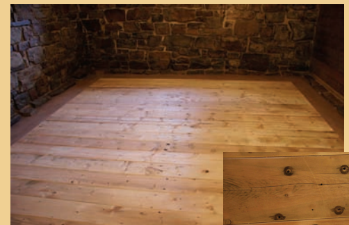
After: Tongue and groove flooring in a Boulder home
