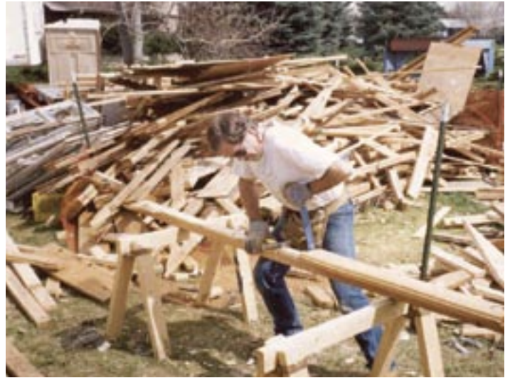
Manual denailing at a deconstruction project.
