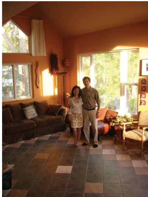
Dark tiles set into a concrete floor capture and store passive solar heat from large south-facing windows at the Marsh home.
